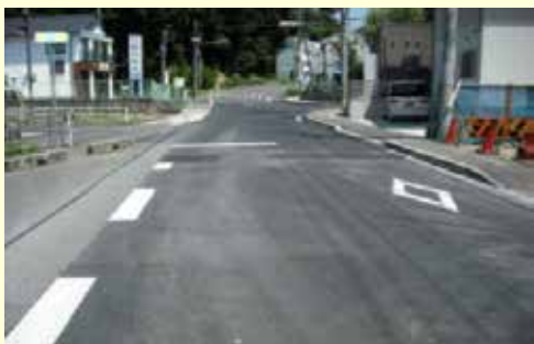
Before execution of the measures
