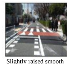
Slightly raised smooth pedestrian crossings
